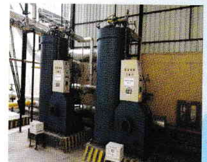
PACKAGED BOILER- 850 KG / HR STEAM
